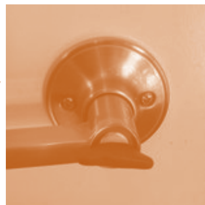
Figure 2: Sugru applied to door lock to make it easier to twist.
