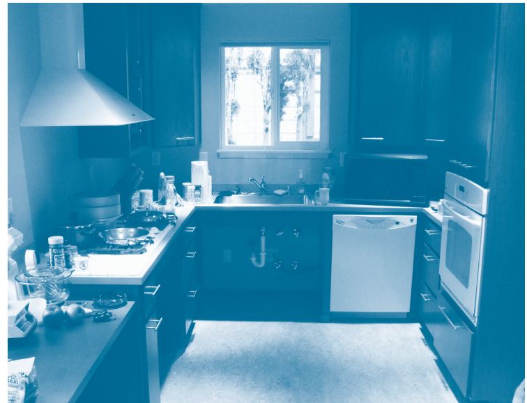
Larry Mohrman’s kitchen was completely torn apart and remodeled to be completely accessible to him. Now he can roll his wheelchair under the stove, sink and counter, and the oven for easy reach. Upper cabinets have pull-down accessible shelf racks. See more photos at http://sci.washington.edu/info/newsletters/articles/12_spr_remodel.asp .
